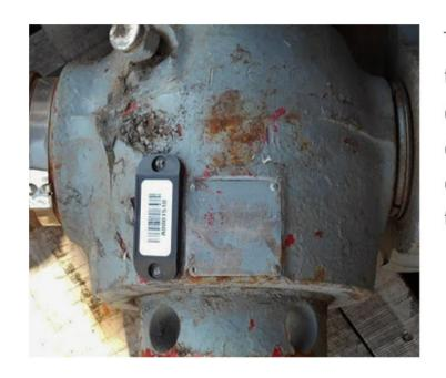
The RFID tag chosen to support the harsh environmental conditions of an oil field was epoxied to the plug valve to ensure the tag survives the life of the asset.
